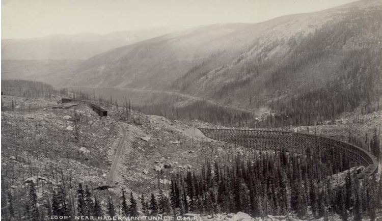
179 HAGERMAN TUNNEL. Hagerman Tinnel, C.M.Ry. ca. 1890. Original photograph, albumen print, 18,6 x 10,6 cm. Photograph no 4. 72,00
