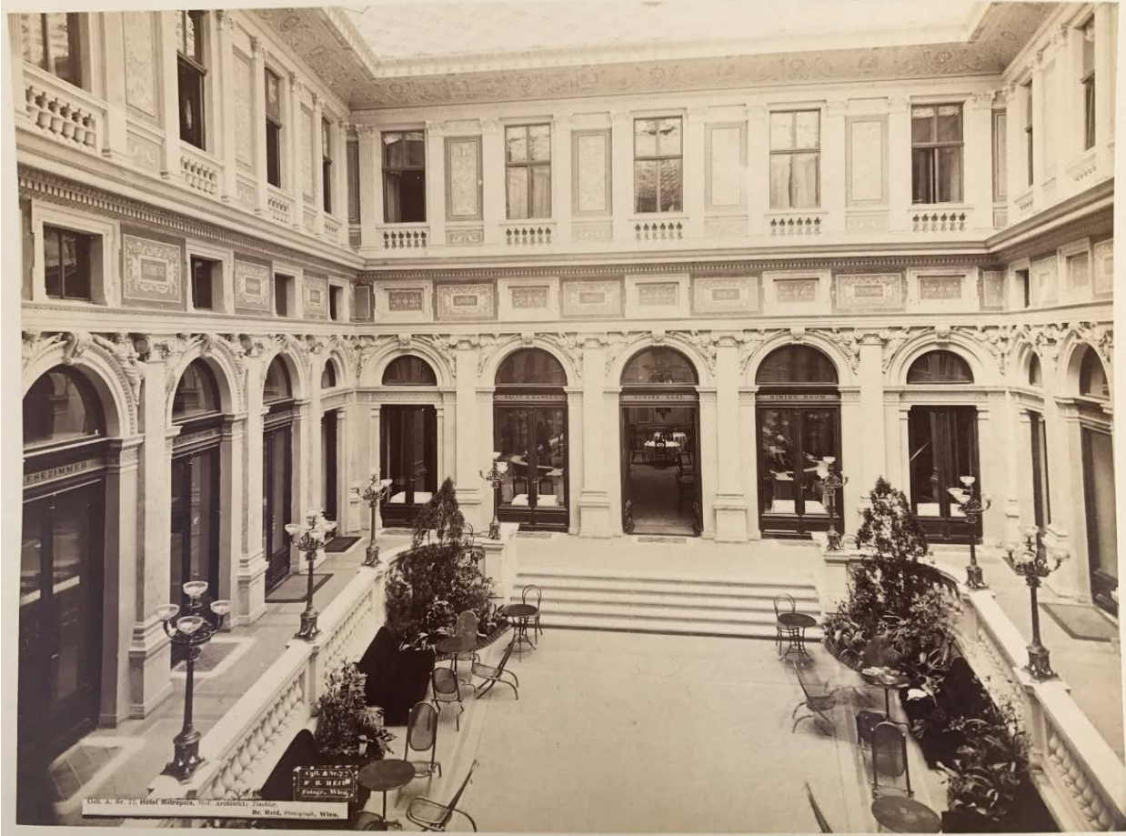
0277 Dr. Hermann Heid, Wien (1834-1891). Hotel Metropole . Vienna: c. 1870. 1 Albumen print. 27 x 20 cm. Mat-boards. Very good.
