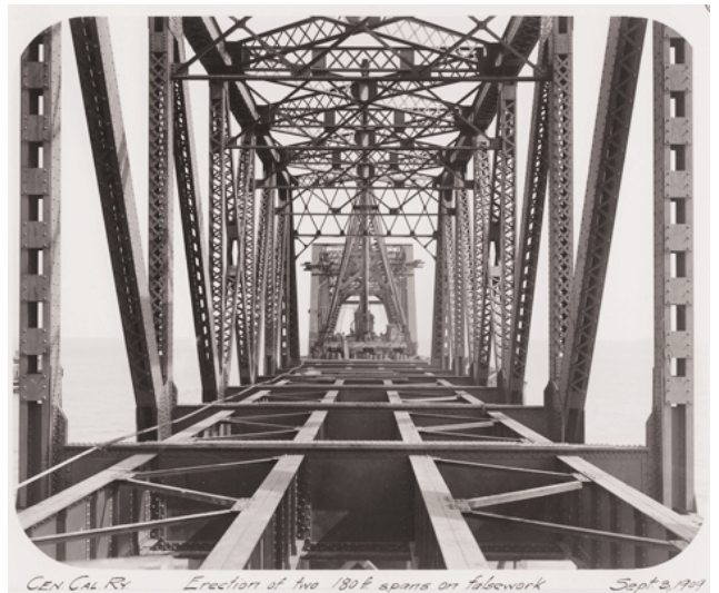
54. CEN CAL RY. Erection of two 130 ft spans on falsework Sept 2, 1909
