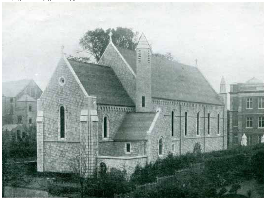
General View of the Exterior of the Chapel.
