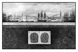
tion of the Thames tunnel, the first known tunnel to have successfully been built underneath a river. The illustrations include architectural plans and engineering diagrams for the project, as well as a frontispiece showing a completed section of tunnel lit with gas lamps. Diagrams also demonstrate exactly how workers were able to remove earth and lay
