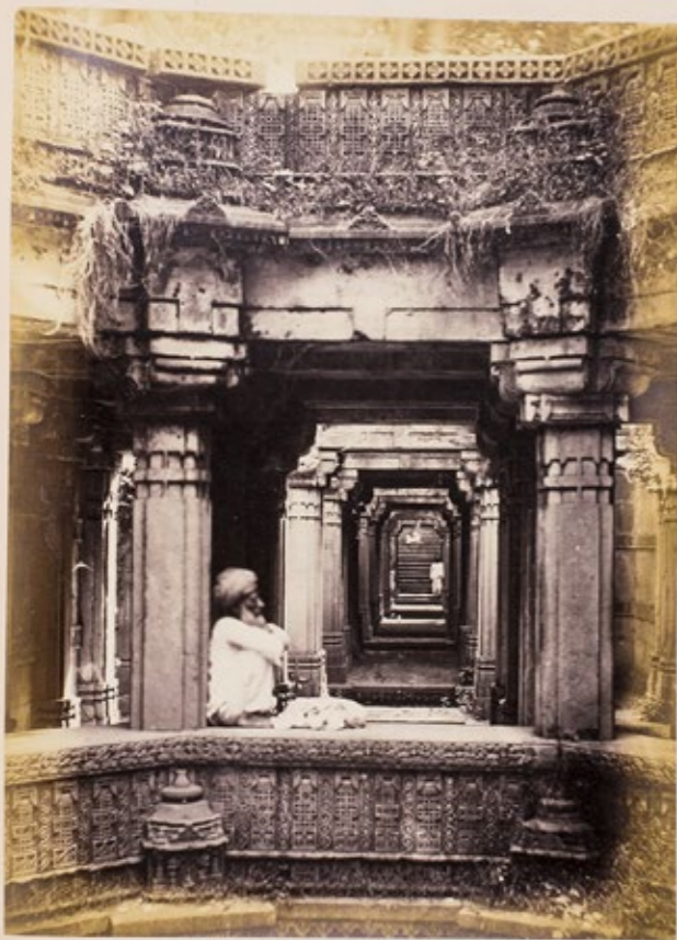
80. DADÁ HUREES WELL AT ASÁRWA.—The upper Gallery.
