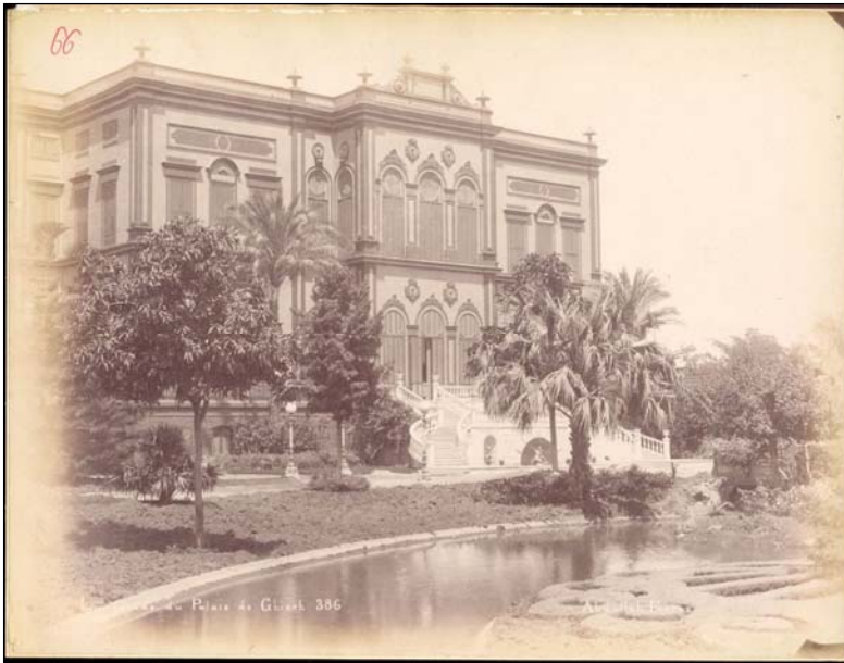
17. ABDULLAH FRÈRES (Abdullah Brothers, Hovsep and Kevork): La facade du Palais de Ghizeh. [Facade of the Palace of Prince Hussein Kamel in Cairo], cca. 1880.
