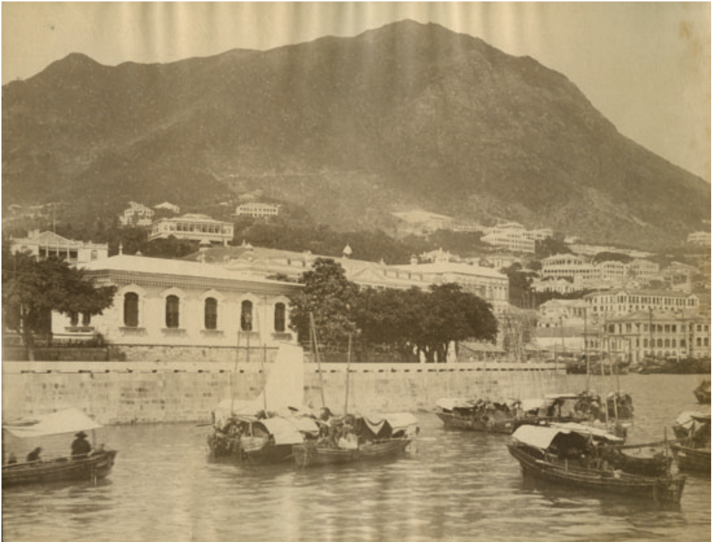
78. Photographer unidentified. The end of Government Pier, showing cricket club, looking towards central, Hong Kong. c.1880. £650
